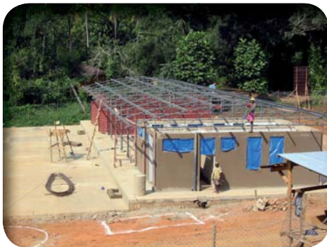
The Tawa market roof under construction (up) and the retail shops alongside the Tawa market plot (right).
